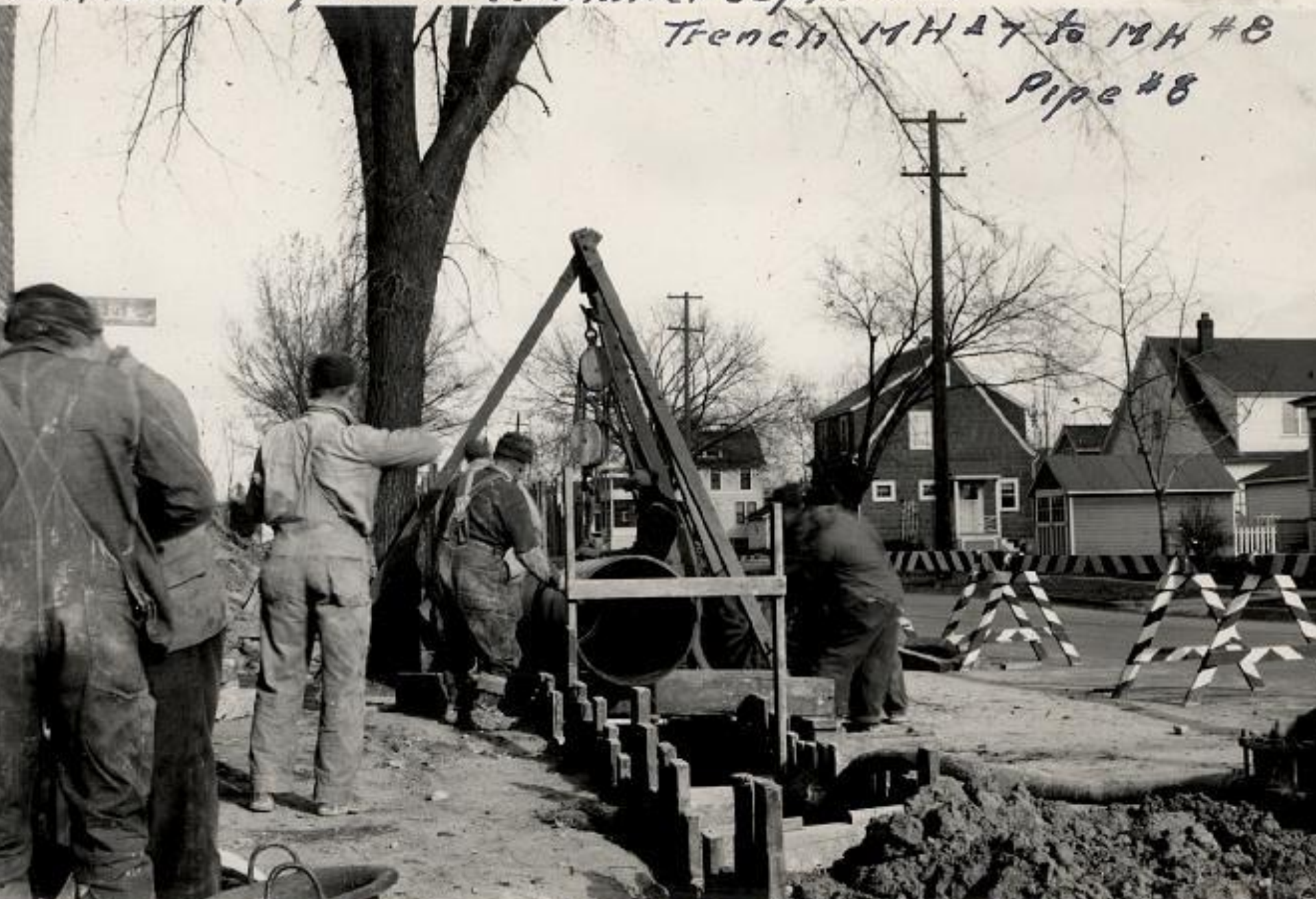
Sling around Pipe... hooked to derrick... setting on timbe
